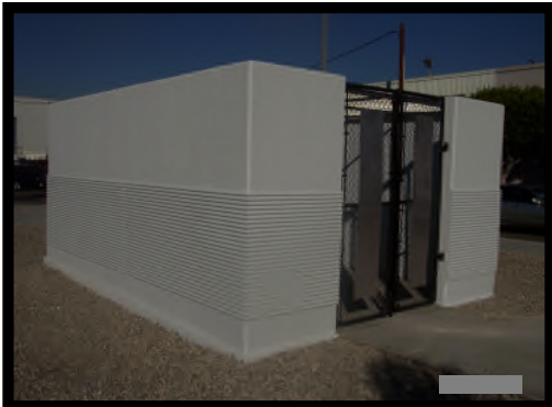
Los Angeles Air Force Base, El Segundo, CA Bldg. 281: Constructed Trash Enclosure With Concrete Pour-In-Place Walls, Foundation Call Henry, Inc. - Jose Perez (310) 597-3323
